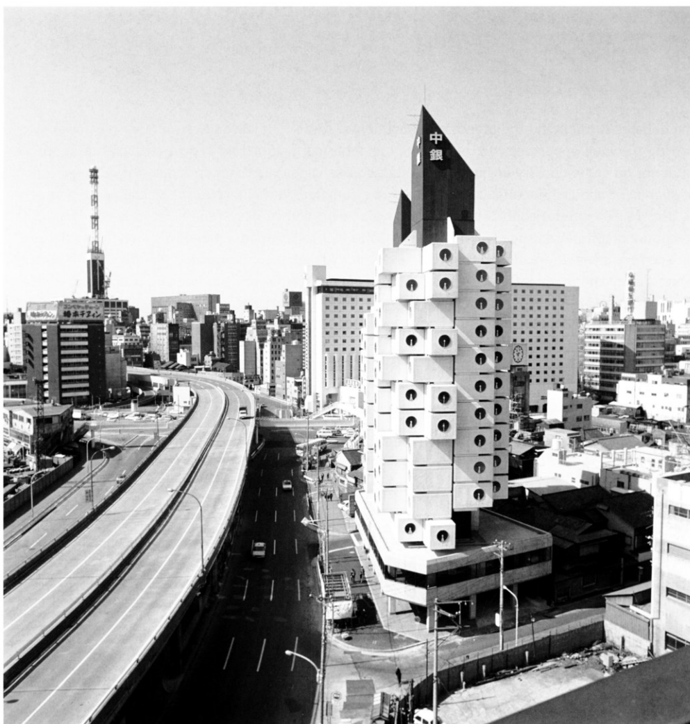
Figure 9: Kisho Kurokawa, Nakagin Capsule Tower, 1972 (Photo courtesy of Kisho Kurokawa Architect & Associates). 85
